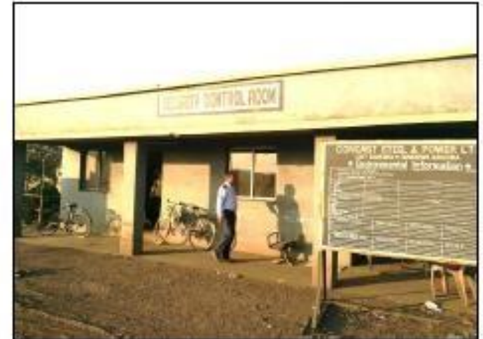
Security Control room
