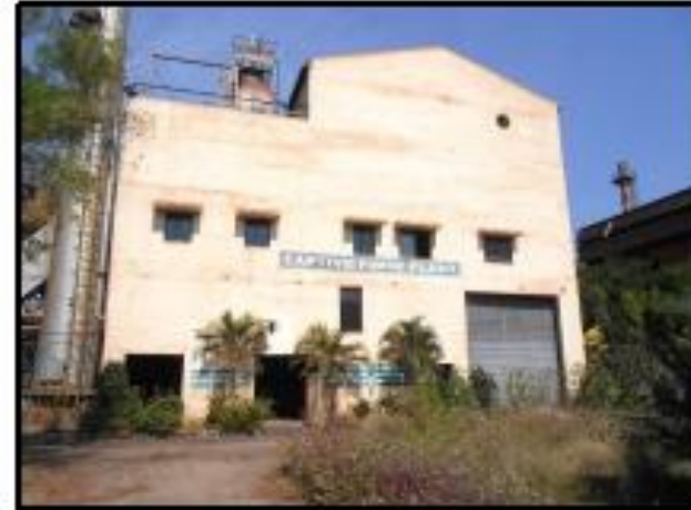
External View of captive power plant.
