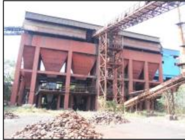
External view of RMH Equipment
