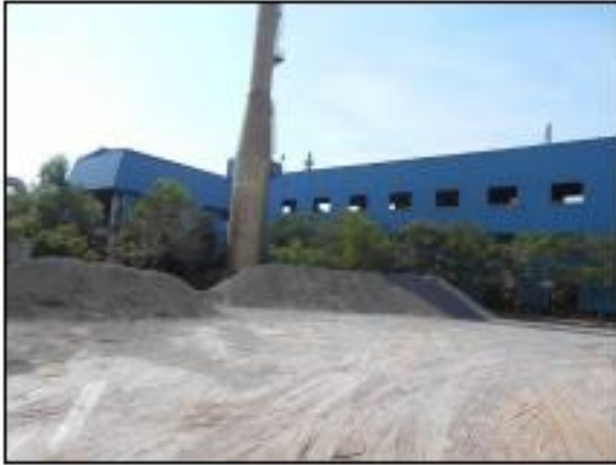
External View of Sinter Plant
