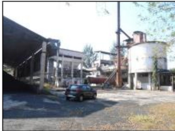
External View of Cement Plant
