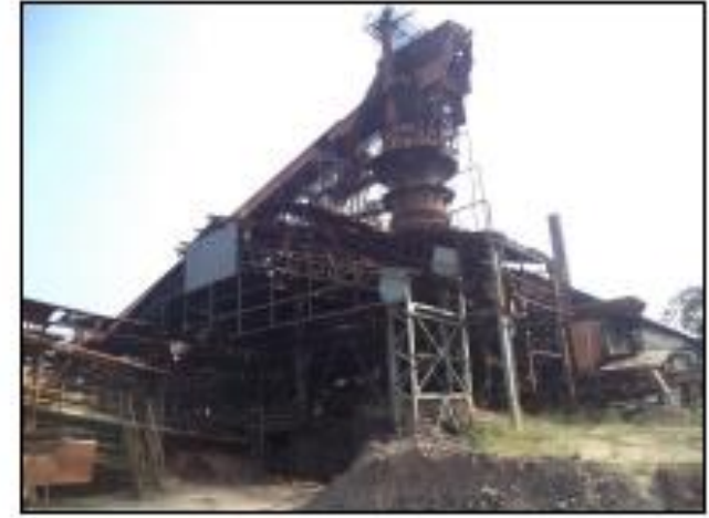
External View of MBF unit
