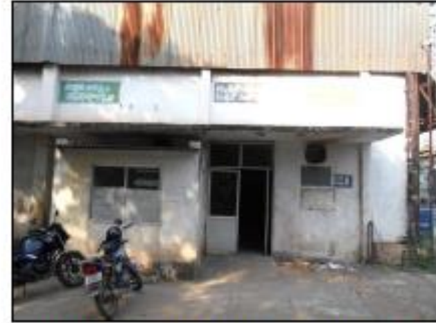
External View of Electrical Control Room
