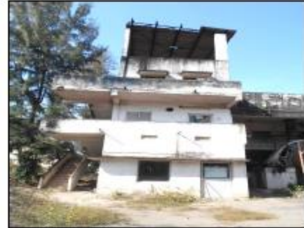
External view of Office at Cement Plant
