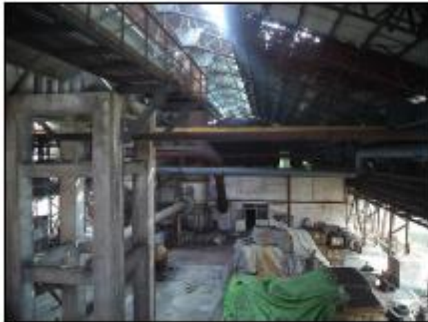
Internal View of MBF unit
