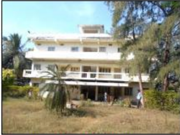
External View of Guest House
