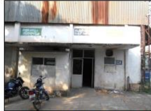
External View of Electrical Control Room
