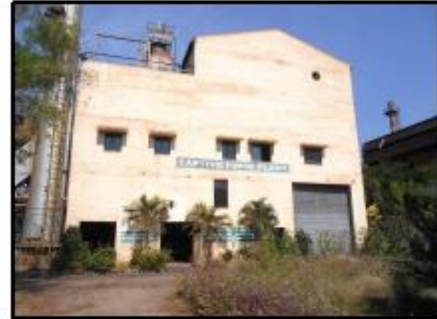
External View of captive power plant.
