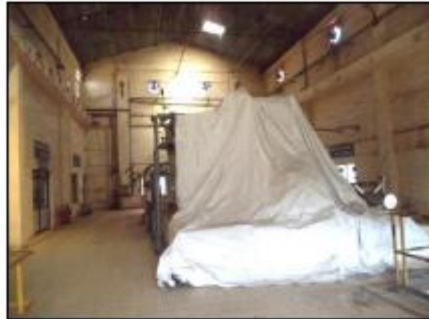
Internal View of captive power plant
