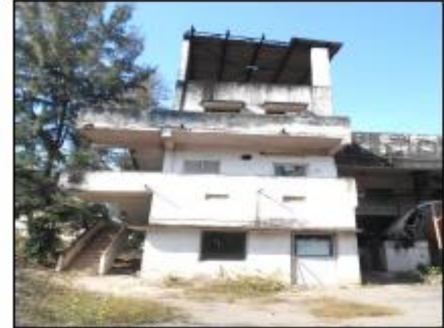
External view of Office at Cement Plant
