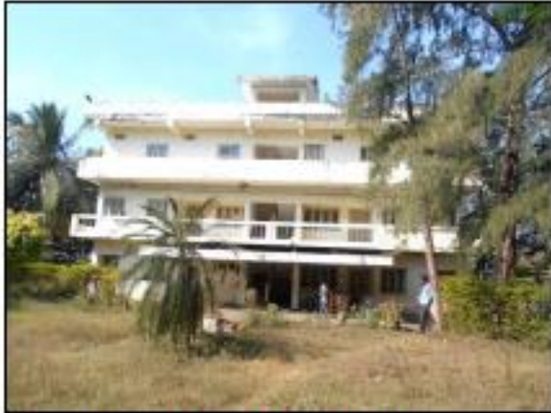
External View of Guest House
