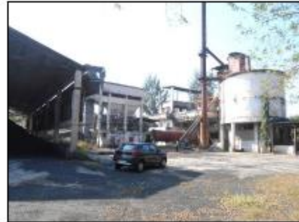
External View of Cement Plant
