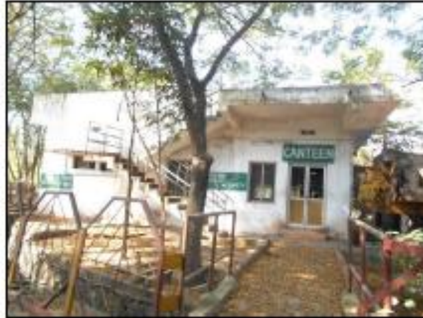
External view of Canteen
