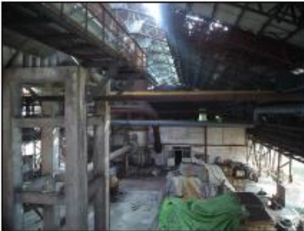
Internal View of MBF unit
